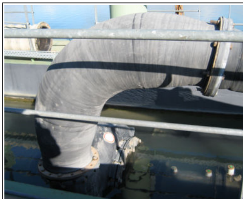
reinforced wear layer for extremely abrasive applications
