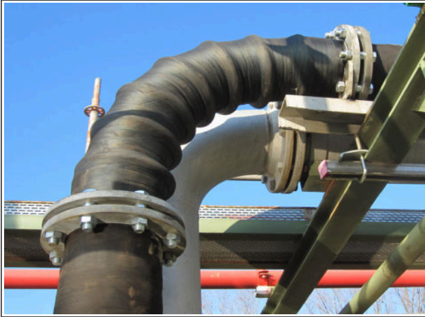
vacuum-proof bend with steel rings
