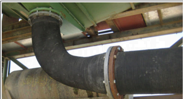
bend with diameter expansion
