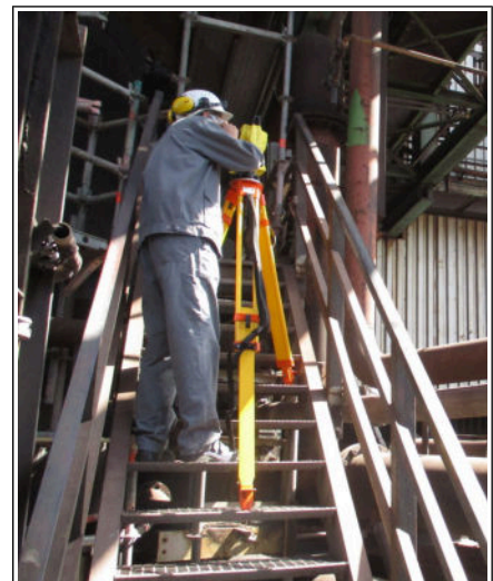
3D survey with total station
