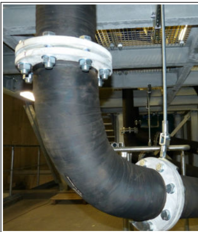
vacuum-proof bend with steel rings
